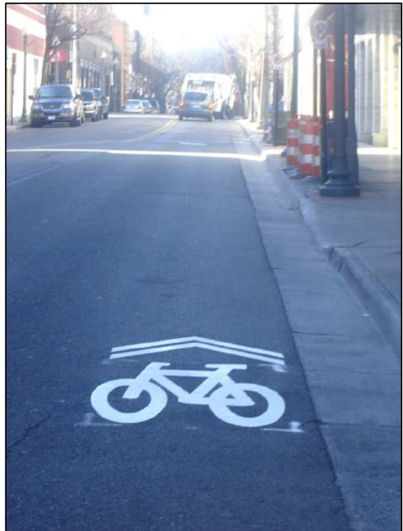
Sharrows (shared lane marking) on Church Street in downtown Roanoke. Markings also serve as wayfinding for on-street bicycle connection between Mill Mountain Greenway and Lick Run Greenway
