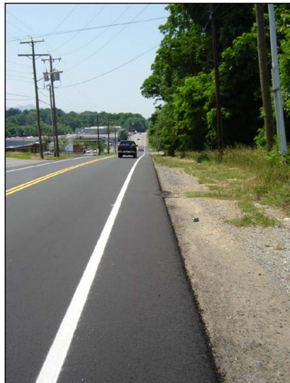
Wide travel lane and paved shoulder on Shenandoah Avenue installed as part of the 2010 annual paving program
