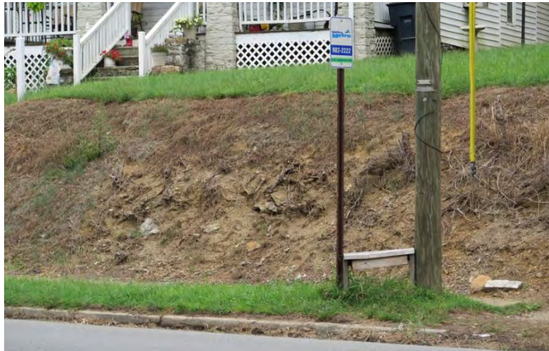
Figure 9: Makeshift pedestrian facilities at bus stops
