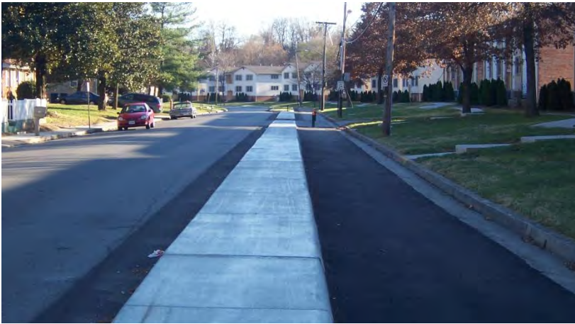
Figure 22: Adding no new impervious surfaces, Westside Boulevard was redesigned to accommodate pedestrians/bikes within the existing street pavement along a path separated from traffic by a concrete median, City of Roanoke
