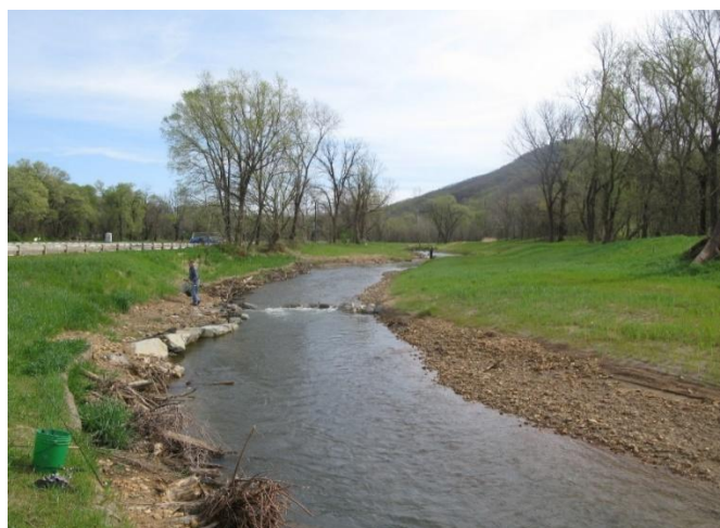
Glade Creek in Vinyard Park after natural stream restoration project. Note provision of floodplain shelf and in-stream structure to lessen erosive stress, and use of toe wood to provide natural habitat.
