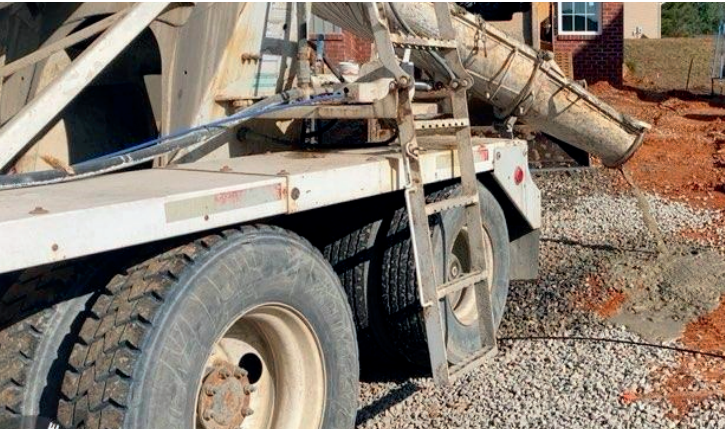
Concrete washout is toxic; it is illegal to openly discharge it.
