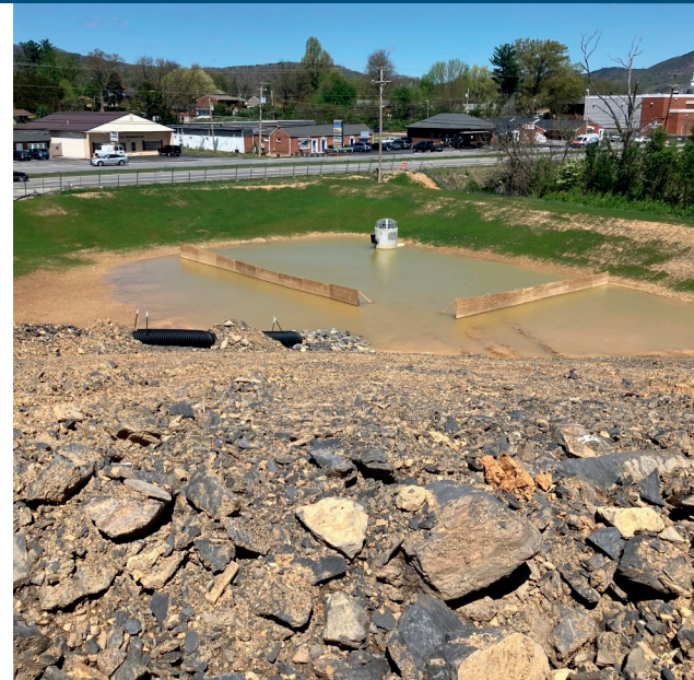
Well-stabilized sediment basin with baffles at the CTE facility.
