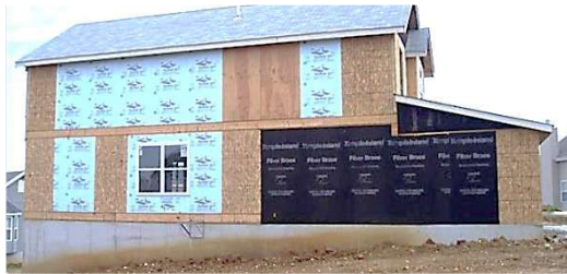
FIGURE 6: INTERMITTENT BRACING
