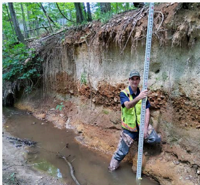
Existing eroding vertical banks in Wolf Creek will be corrected in Phase 2 of this stream restoration project.
