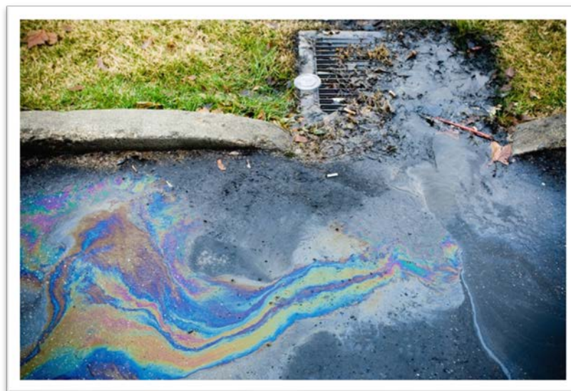
An illicit discharge of oil into the storm drainage system.
