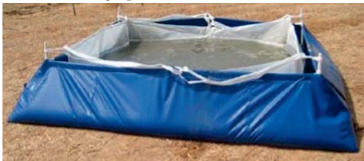
A well-maintained vinyl container for concrete washout. Once these devices become full, they must be replaced, if still needed. Photo: courtesy of US EPA.
