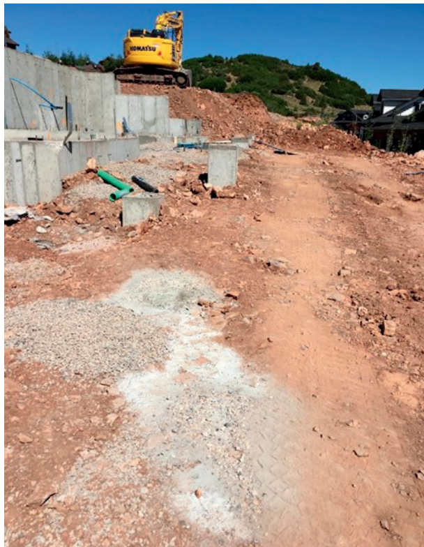
Concrete wash water residue from improper washout onto ground. Photo: courtesy of Michelle Donohoe, Roanoke County.
