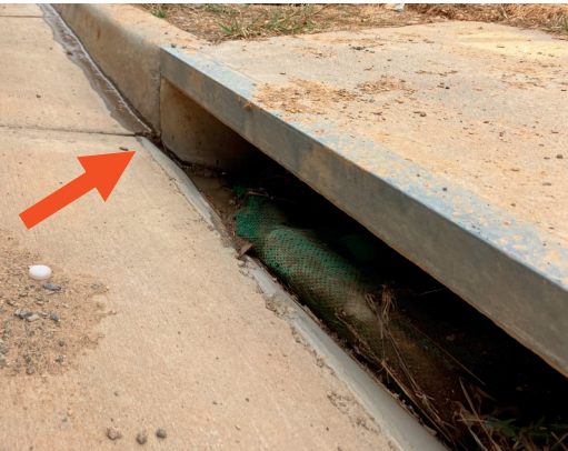
Illicit discharge (concrete washout) entering an unprotected curb inlet. Be sure to provide and maintain proper inlet protection.
