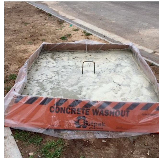
A prefabricated cardboard concrete washout, by Outpak. Photo: courtesy of Construction Washout. https://www.constructionwashout.com/
