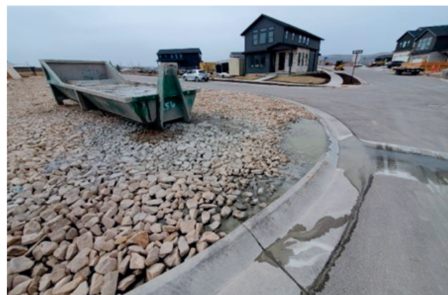
Toxic concrete washout from an overflowing roll-off container. Photo: courtesy of Michelle Donohoe, Roanoke County.
