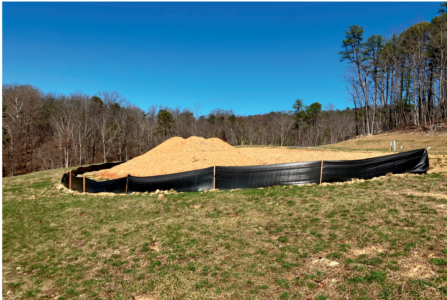
Properly entrenched silt fence serves as an excellent sediment control device around soil stockpiles and project perimeters, which protects downstream waterways.
