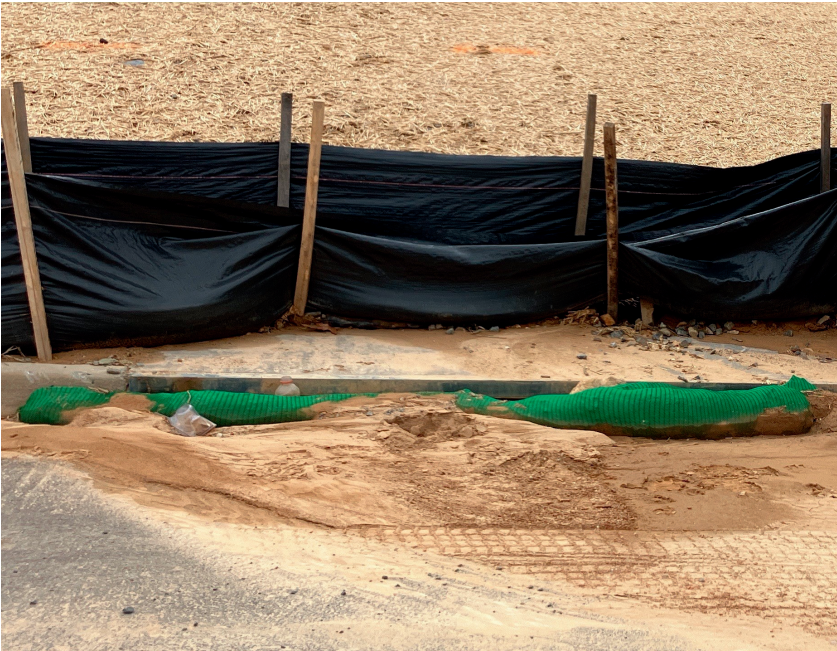
Illicit discharge (sediment) onto street and into drainage inlet. Be sure to remove sediment when it reaches 1/2 the height of the inlet protection device. Ensure to sweep the street at the end of every work day.
