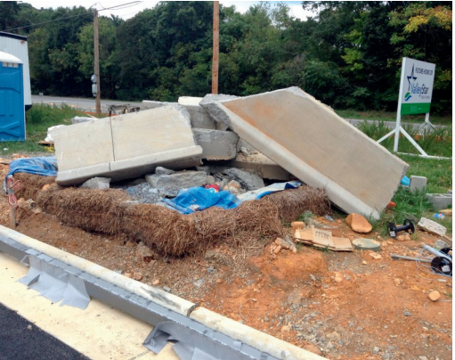
This concrete washout is full and unusable. Make sure concrete washouts are accessible for use and replaced as needed.
