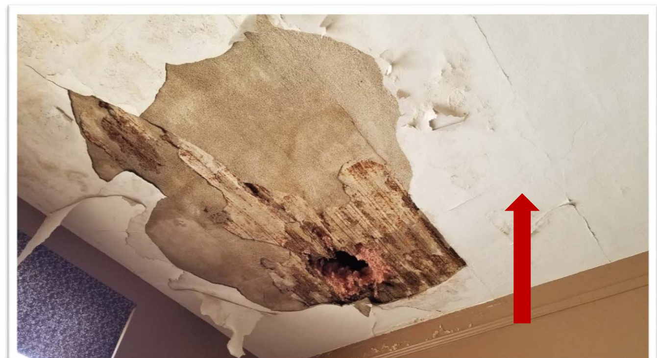
Photograph #0026 (1930) HA 6 – 2 layer plaster ceiling with asbestos in base coat (Trace <1% Chrysotile)
