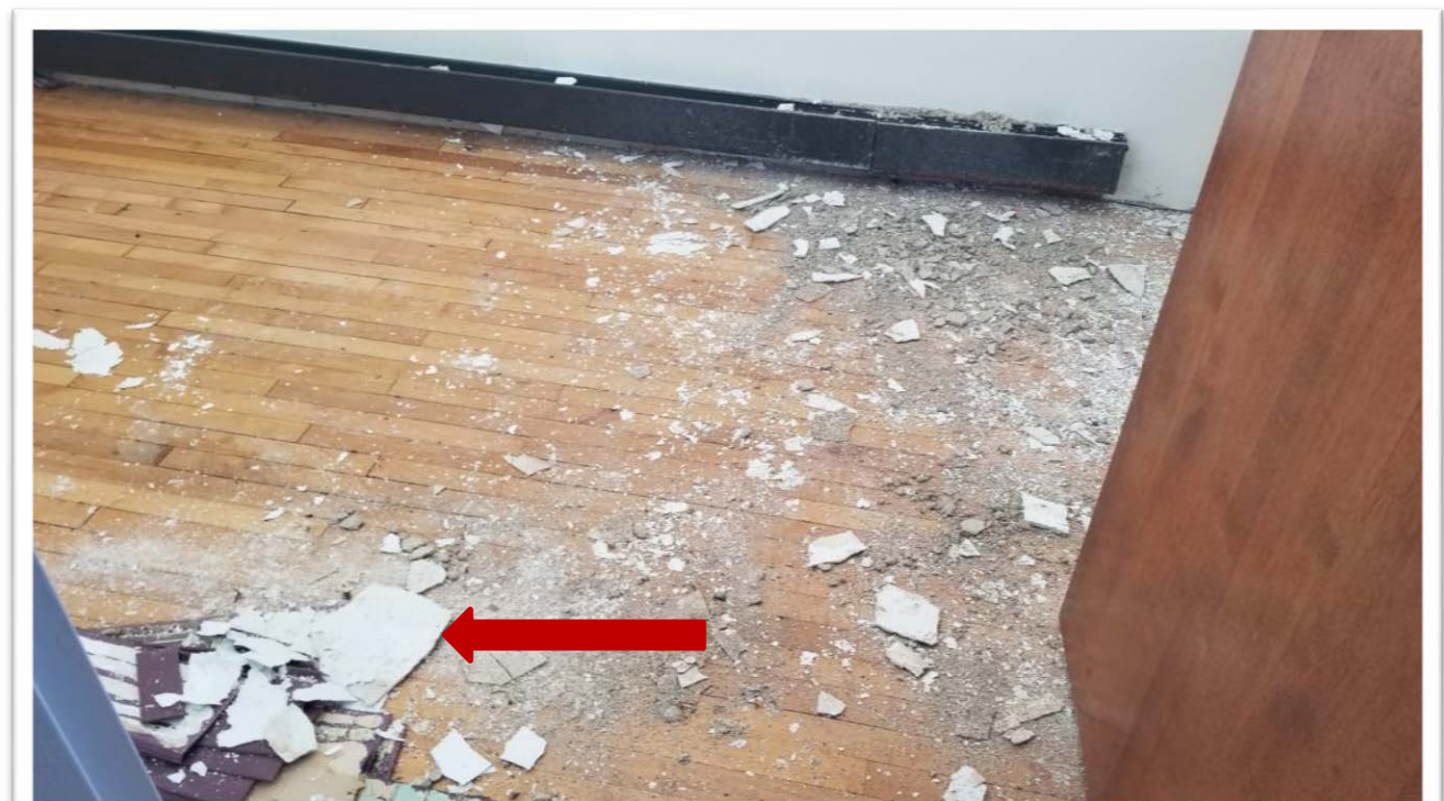
Photograph #0024 (1930) HA 6 – Damaged 2 layer plaster ceiling with asbestos in base coat (Trace <1% Chrysotile)
