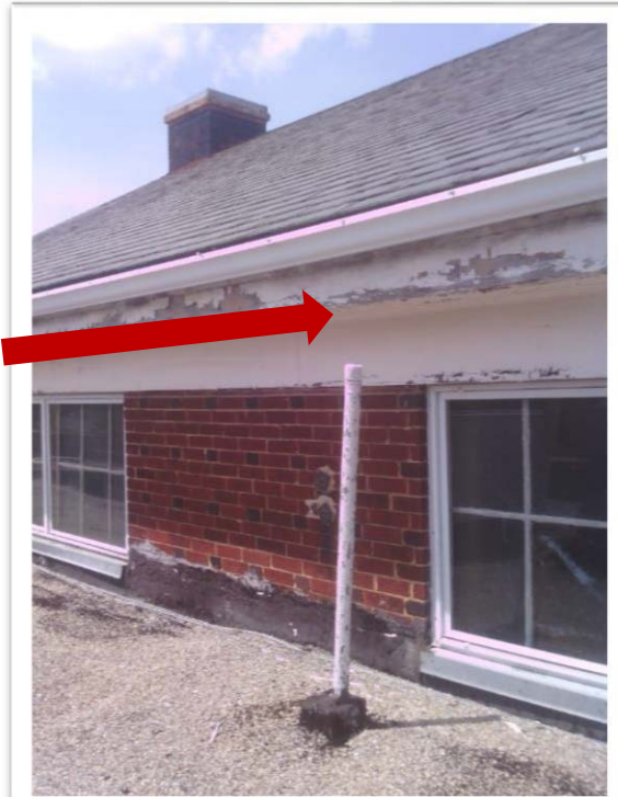
Photograph #0035 Lead Based Paint on roof trim on 1930s building
