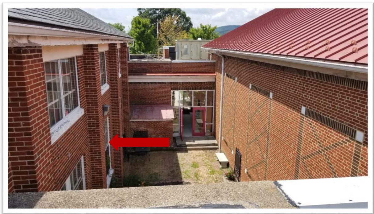
Photograph #0023 (1930) HA 5 – Exterior window with multiple caulk layers containing asbestos: (Trace <1% Chrysotile, 3% Chrysotile); presumed ACM on upper windows.
