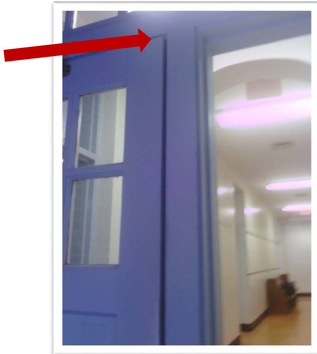
Photograph #0033 Lead Based Paint on door casing and transom
