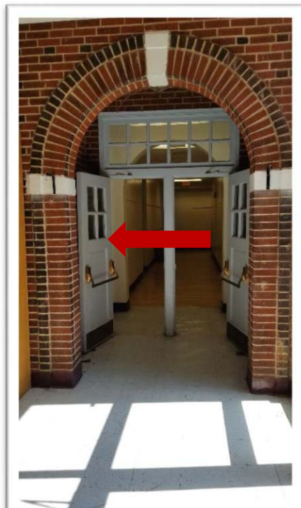
Photograph #0021 (1930) HA 3 (Representative Sampling Location) – Double doors with multi-layer caulk on door casing/brick interface containing asbestos (3% Chrysotile)
