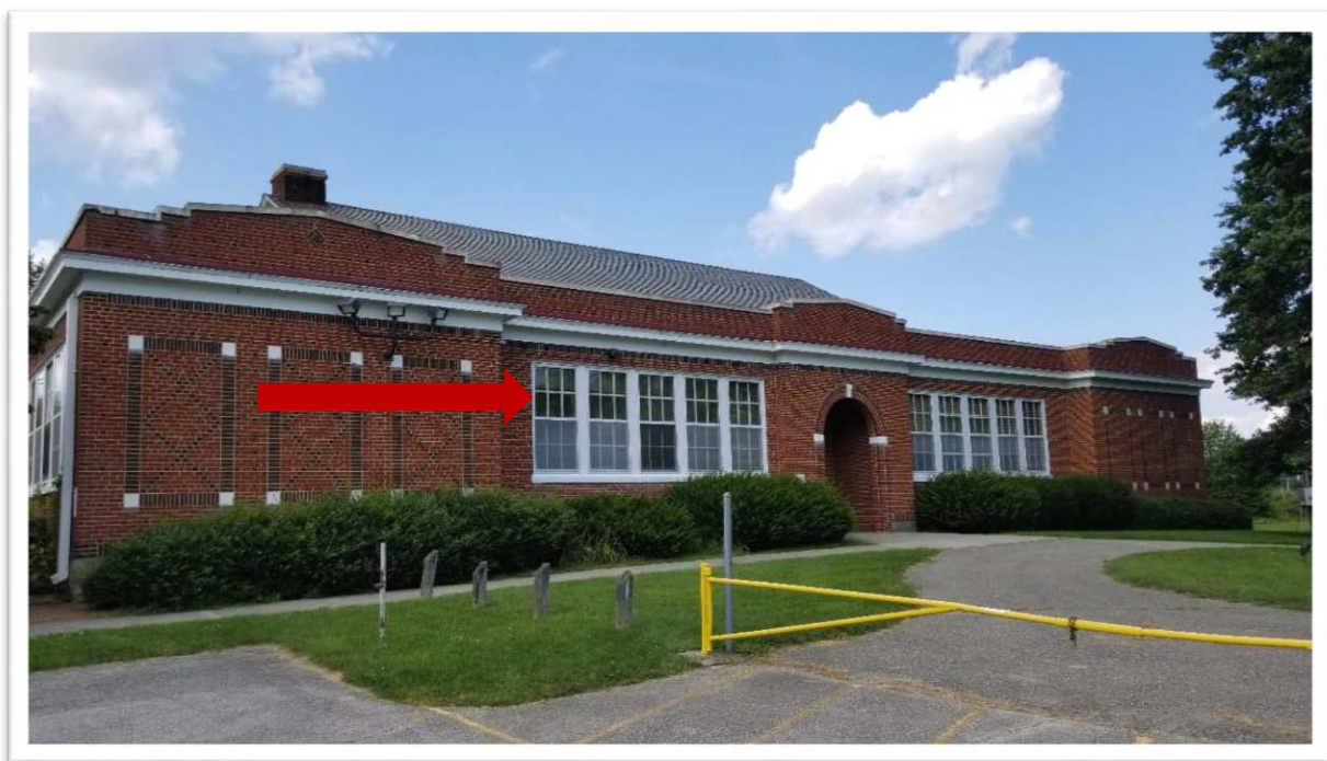
Photograph #0021 (1930) HA 3 (Representative Sampling Location) – Double doors with multi-layer caulk on door casing/brick interface containing asbestos (3% Chrysotile)
