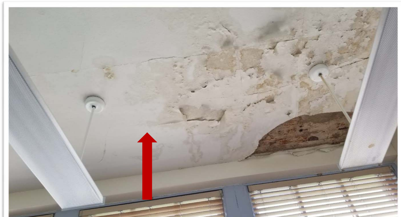
Photograph #0025 (1930) HA 6 – 2 layer plaster ceiling with asbestos in base coat (Trace <1% Chrysotile)
