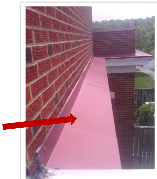
Photograph #0036 Lead Based Paint on roof flashing "awning" on breezeway
