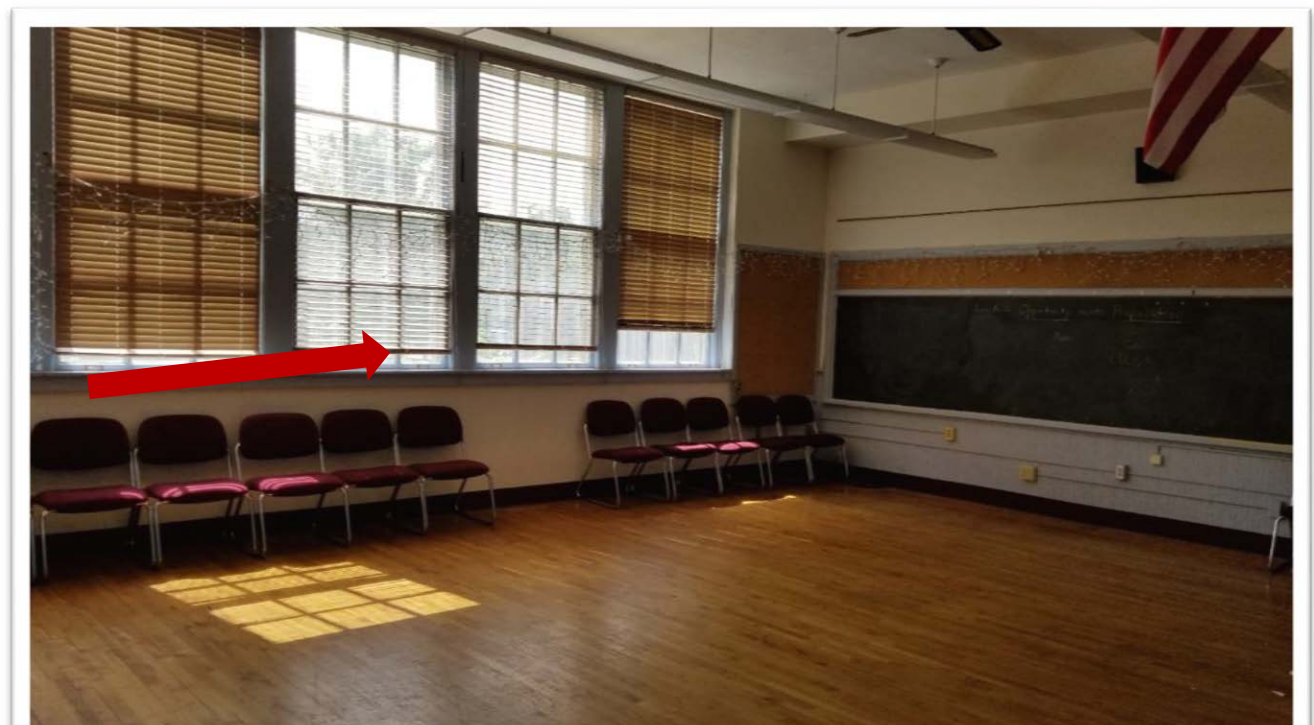
Photograph #0034 Lead Based Paint on window components
