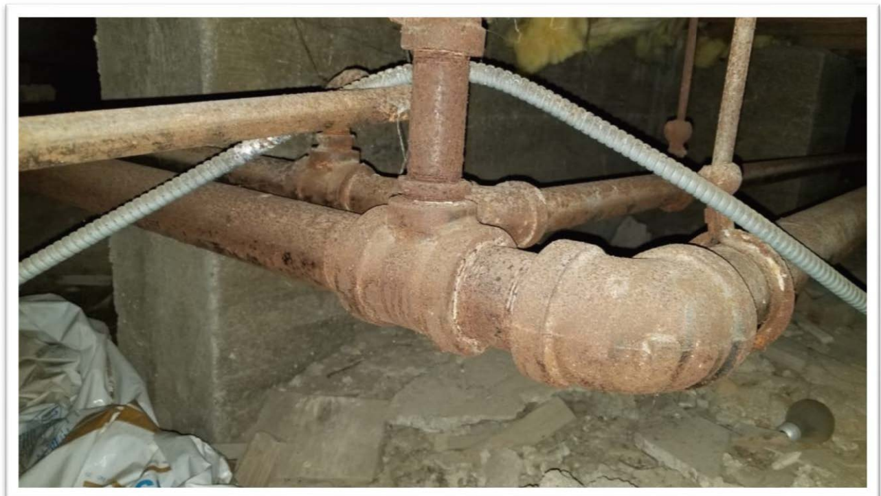
Photograph #0014 1930s crawl space conditions (uninsulated pipe)
