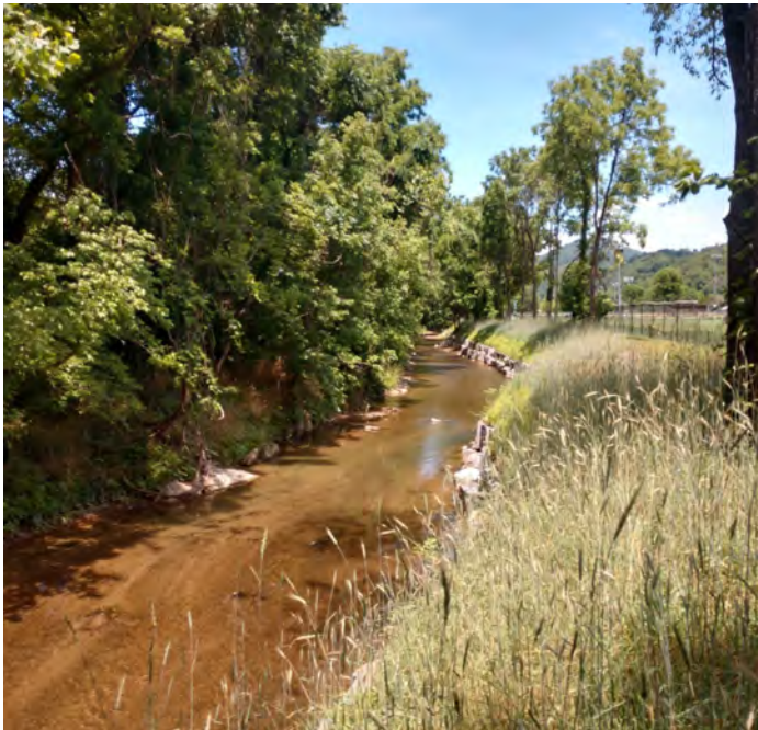
Above: Glade Creek Stream Restoration Project.
