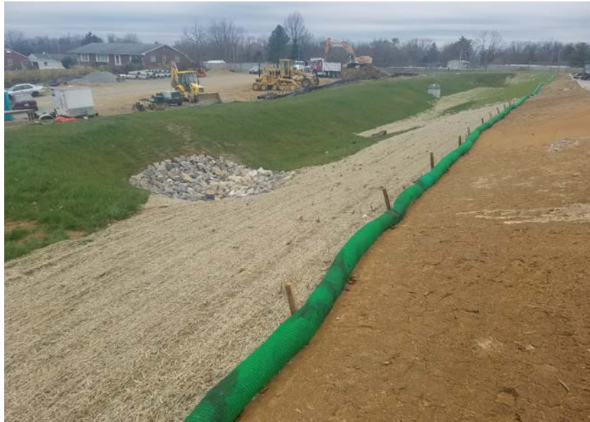
Effective use of erosion control matting and slope interrupters at Parkside Storage
