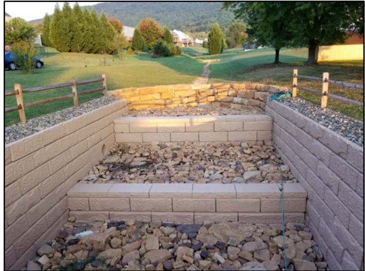
Striking channel improvements in The Orchards subdivision, installed by Stormwater Operations Division, Dept. of Community Development
